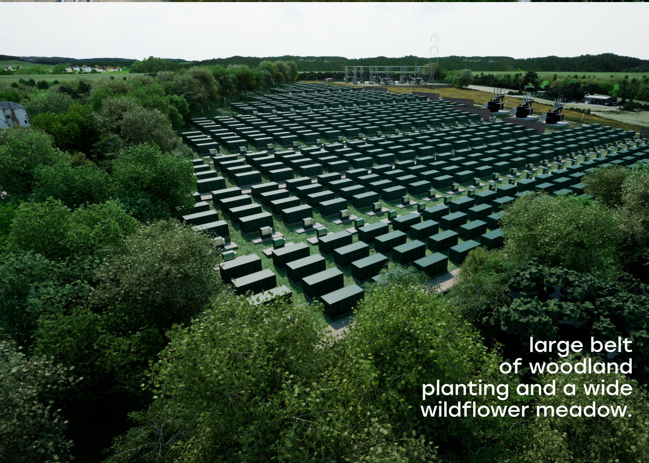
500MW battery energy storage facility
